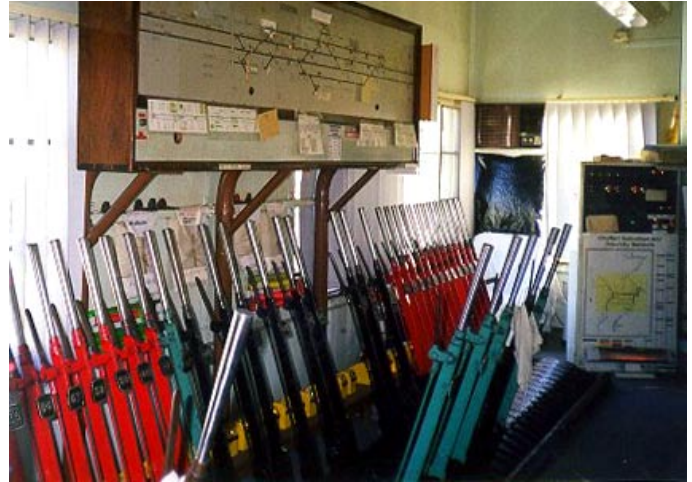
Much of the signalling control technology used in the greater metropolitan region is now extremely dated and offers few of the capabilities available with modern systems. (The mechanical and electric relay-based systems shown here, at Gosford (above), Sefton (below) and Strathfield (left), date back to the early 1900s, the 1920s and the 1970s.) The equipment and facilities stand in stark contrast to the modern equipment and high-quality facilities used for monitoring and controlling road traffic flows in Sydney, even though the road monitoring and control systems are not primarily concerned with safety.
